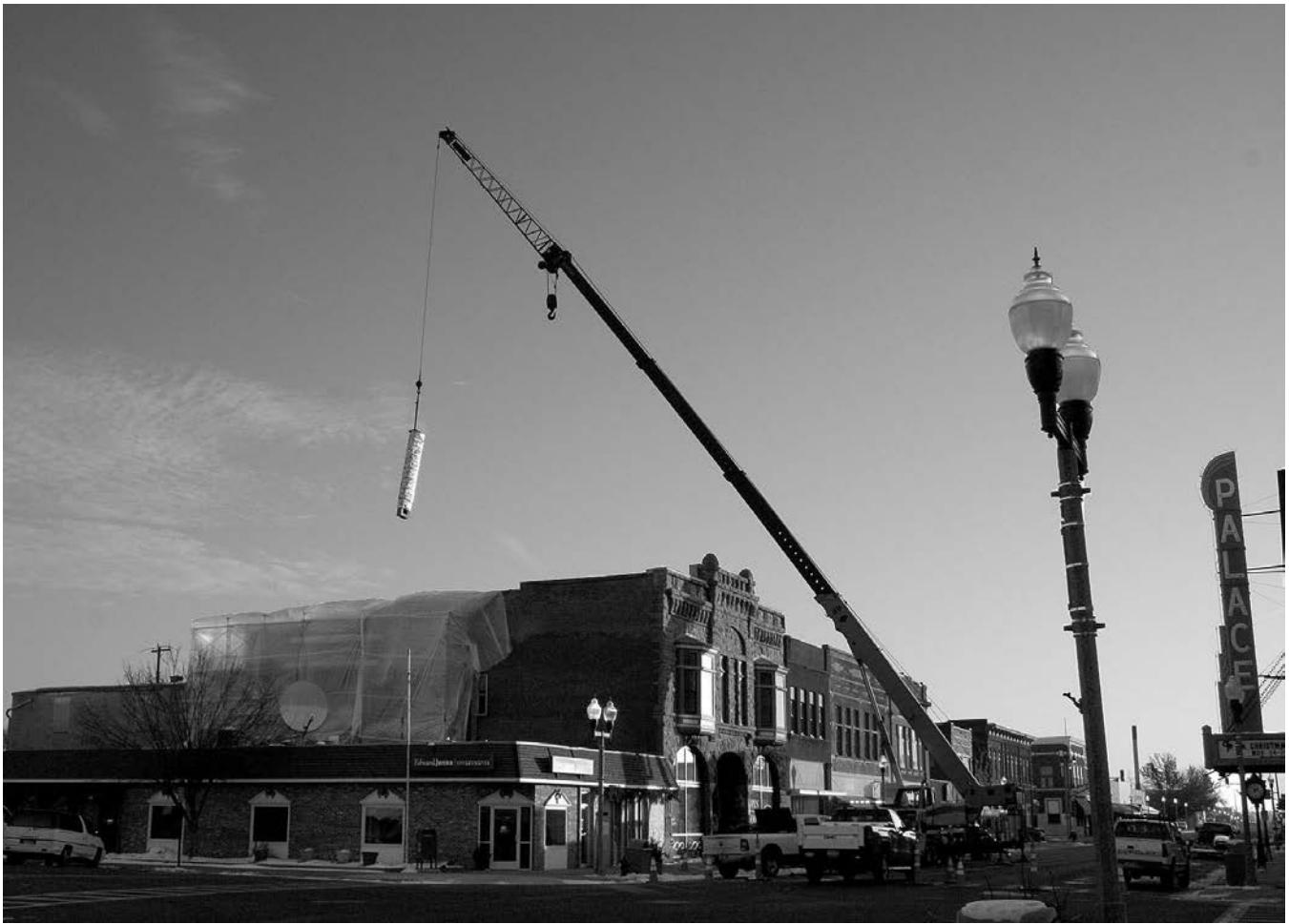
Chantel Connell photo/1126 sterlings crane drops kithcn hood through roof
