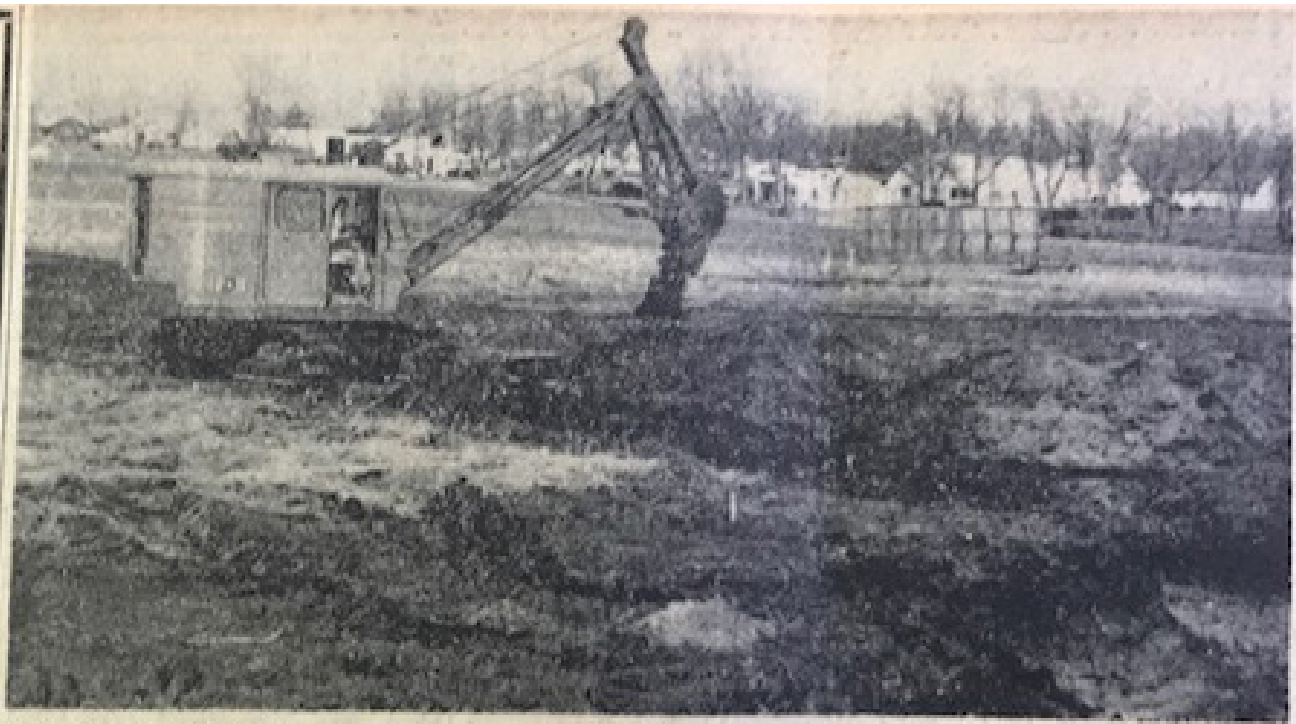
DIGGING OPERATIONS are now in progress at the site of the Laverne junior-senior high school. This power shovel is digging trenches for the foundations of the new building. (Star-Herald photo.)
